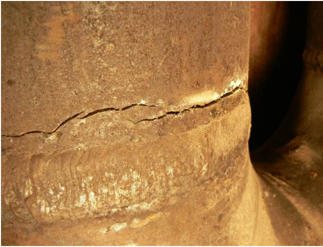
Figure 14. Cracking of the outlet 304 stainless steel tubes in the trim heater
