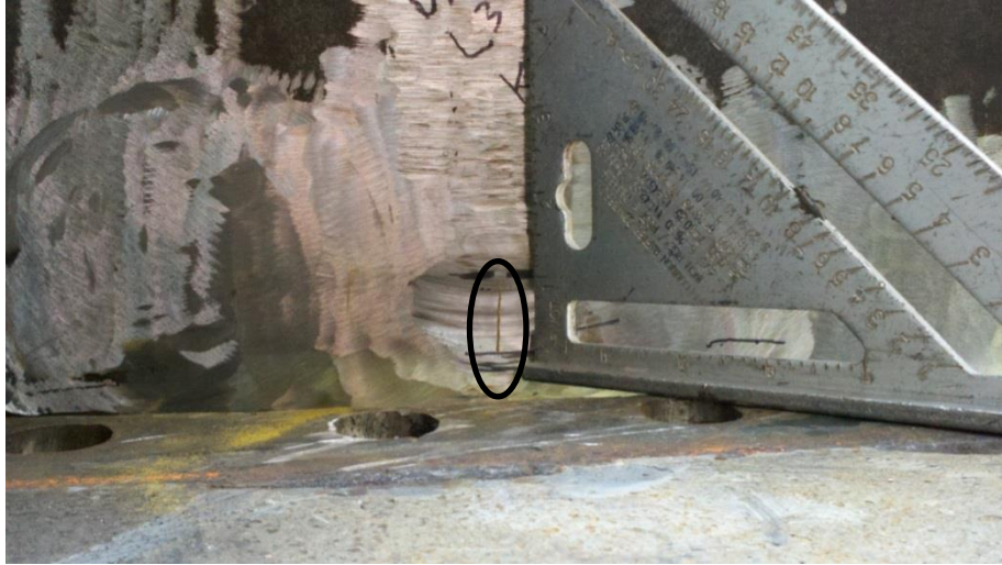
Figure 1-2: Vertical crack located in the SMB arch tie butt weld.
